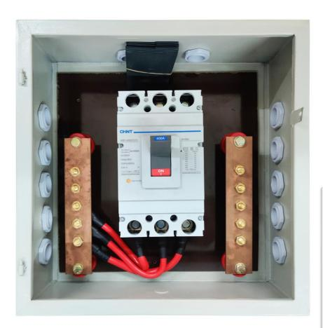
**BusBar for 3 inverters in parallel**
